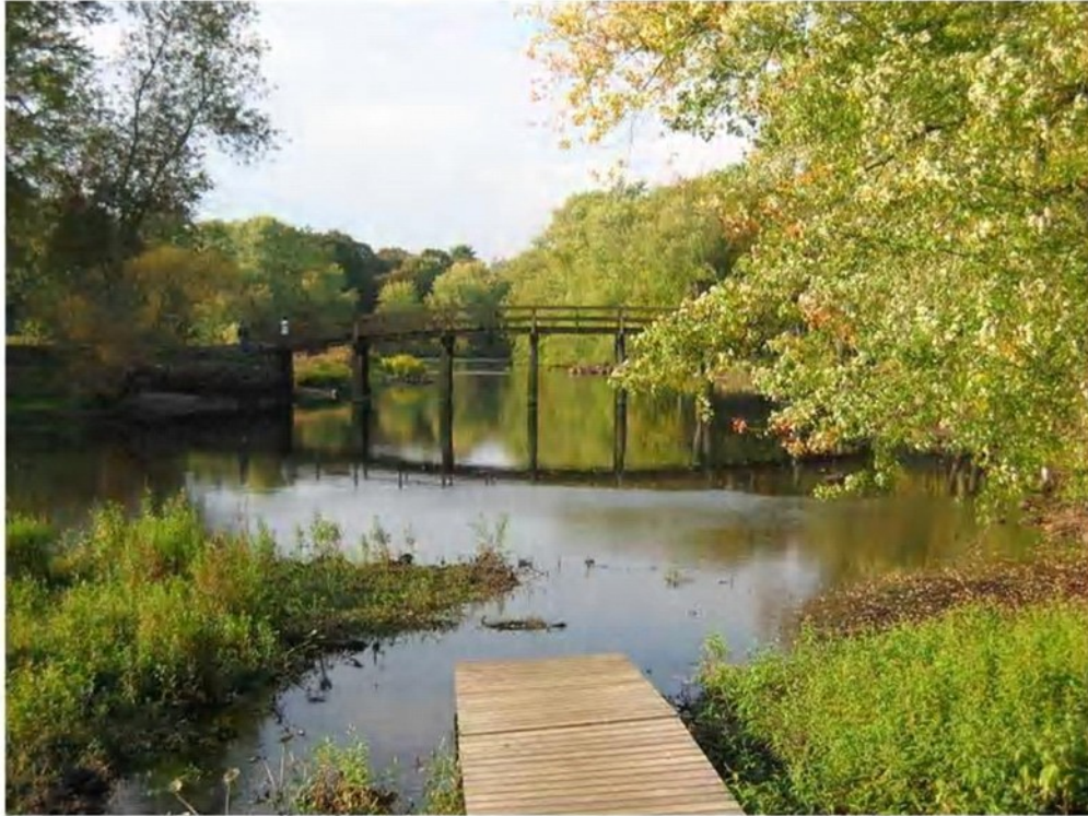
The British Regulars were after reported weapon & ammo stashes spread around the rural areas. The British were thrown back at this bridge.
